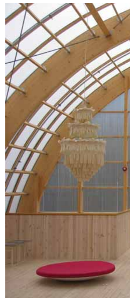
DackeStop Museum of Arts in Virserum, Sweden, using Lexan Thermoclick sheet for its roofing and walls
